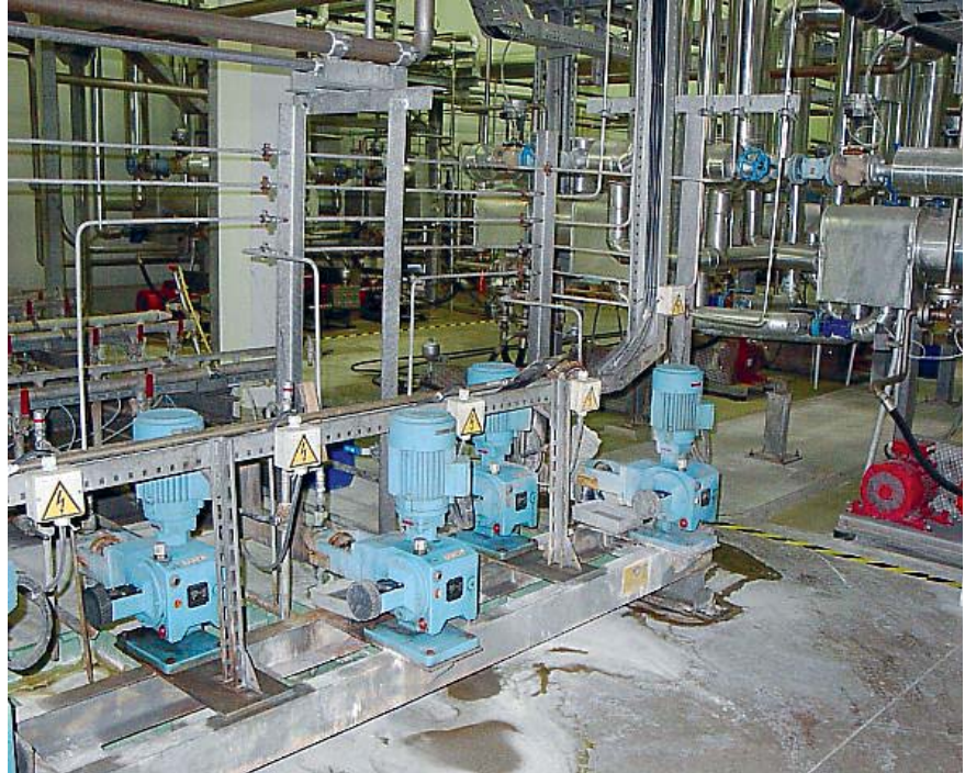
LEWA metering pumps in demanding use for industrial high pressure cleaning
